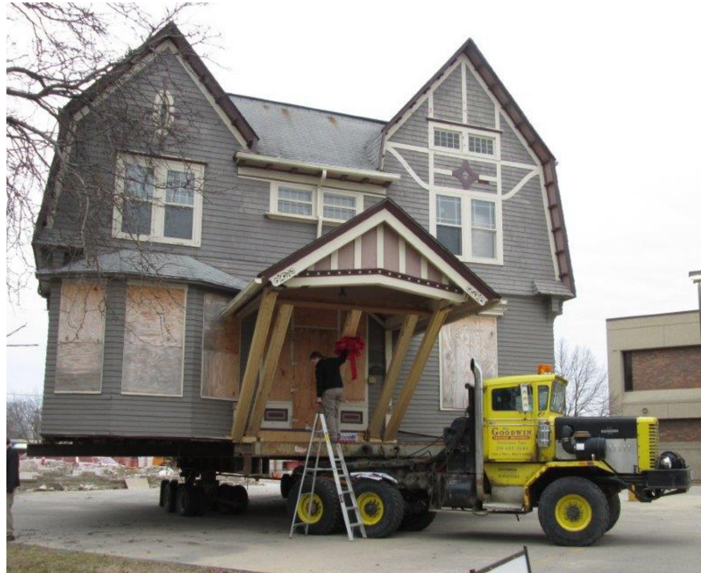
Cultural resources When buildings cannot remain on site, moving buildings can serve as a good alternative for preservation.
